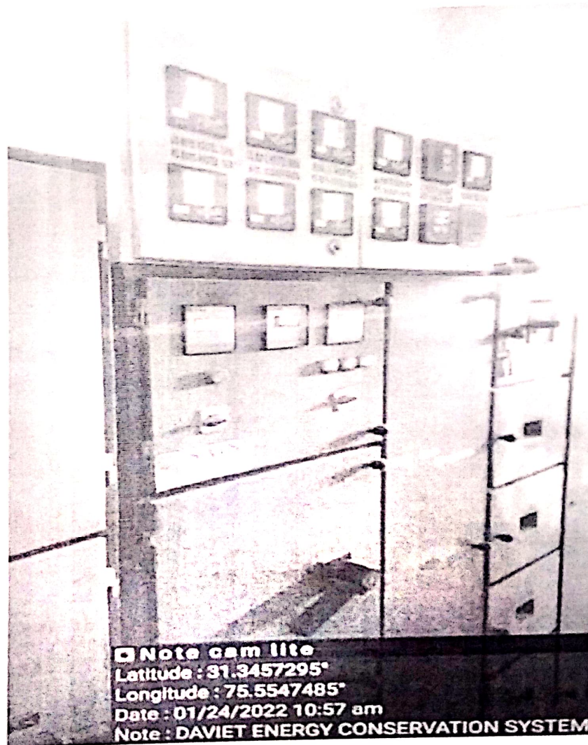
MFM Schneider Smart meter for the Sensor based energy conservation systems (3 no.) installed in DAVIET, Jalandhar
