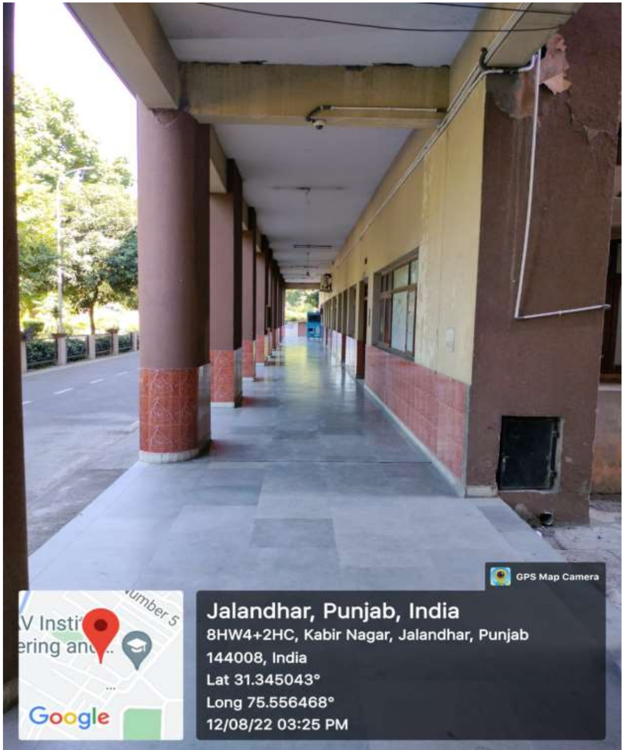
Security Camera in Corridor
